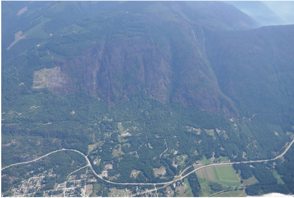
Figure 4. Overview of the Ponderosa FSR face including the drainages to the north of the O'Shea Creek (Photo: T. Giles, SNT Geotechnical).
