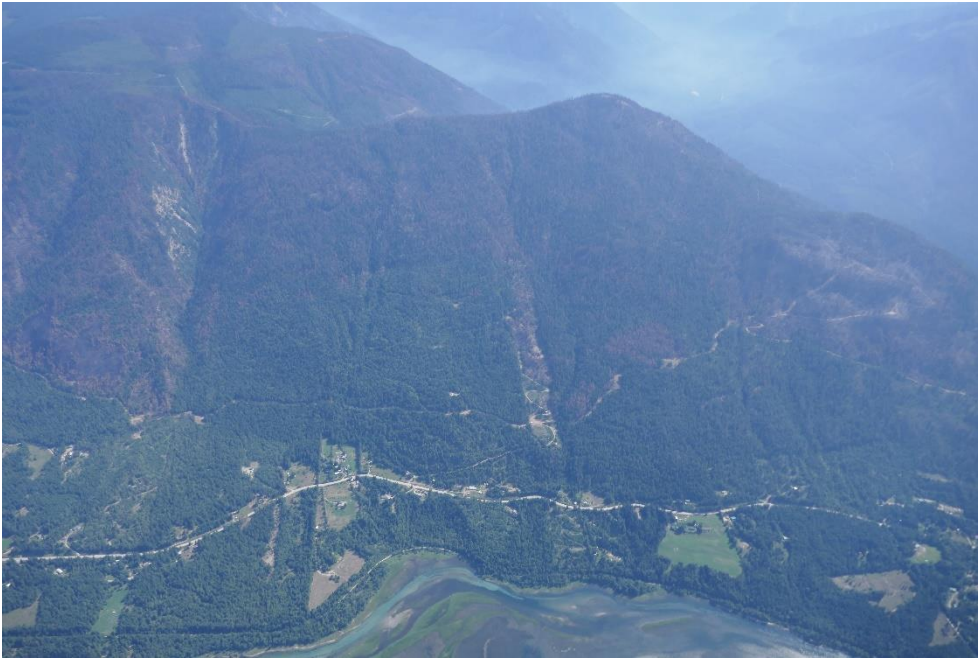
Figure 3. Overview of the Ponderosa FSR face including O'Shea Creek and Ringrose Creek (Photo: T. Giles, SNT Geotechnical).
